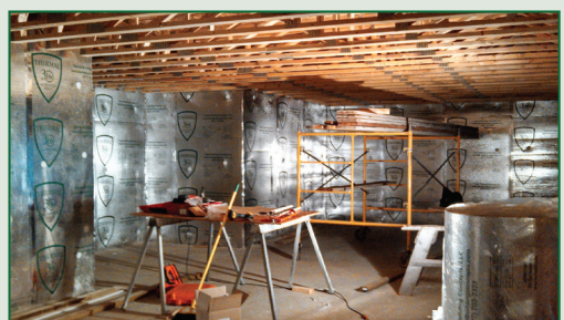
½" RRE Thermal 3Ht installed on exterior walls to complete insulation envelope.
