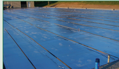
½" RRE Thermal 3Ht insulation placed under concrete slab. Optional to use WRE Thermal 3Ht.
