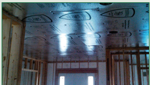
1" RRE Thermal 3Ht installed on exterior basement walls with plastic masonry fasteners.
